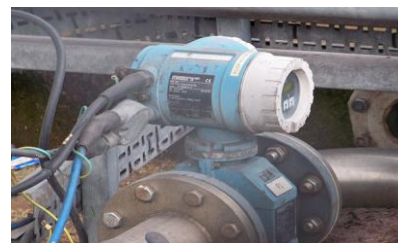
Fig. 8 A magnetic flow meter at the compressor house of an automotive chassis assembly line.
