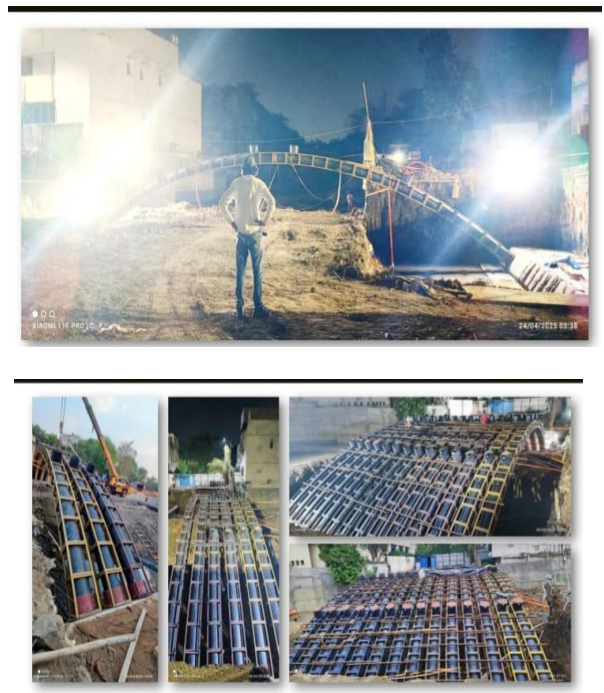
Fig.1: Construction of PowerArch ® Bridge
