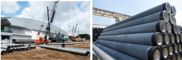
Fig. 6. Pre-stressed Concrete spun pile PHC at the site.
