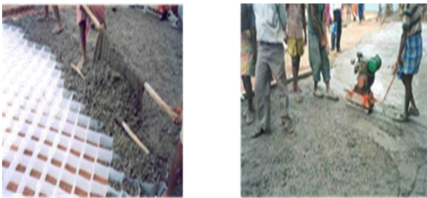
Fig 5 Cell filled pavement under construction and compaction of concrete [4]
