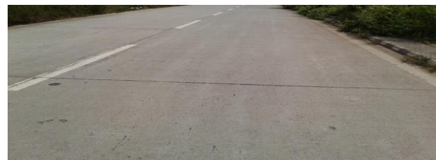
Fig 4 Finished whitetopped pavement
