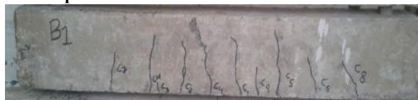
Figure 2: Cracking Pattern of Beam B1/M25/AST1/NF
