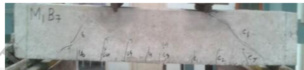
Figure 8: Cracking Pattern of Beam B7/M25/AST2/WF/1%
