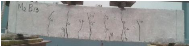
Figure 14: Cracking Pattern of Beam B13/M50/AST1/WF/1%
