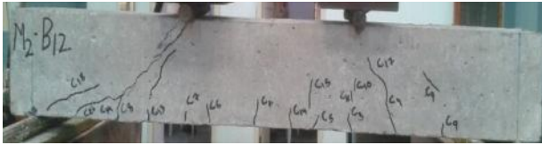
Figure 13: Cracking Pattern of Beam B12/M50/Ast2/Nf
