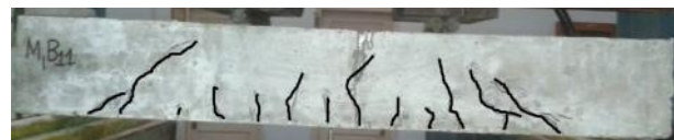
Figure 12: Cracking Pattern of Beam B11/M50/AST2/NF
