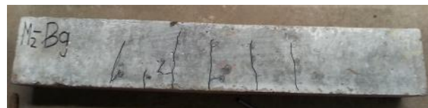
Figure 10: Cracking Pattern of Beam B9/M50/AST1/NF
