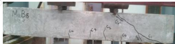
Figure 9: Cracking Pattern of Beam B8/M25/AST2/WF/1.5%
