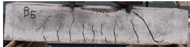
Figure 6: Cracking Pattern of Beam B5/M25/AST1/WF/1%
