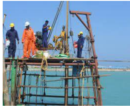
Fig. 2. Offshore geotechnical investigation
