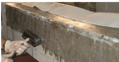
Fig 4 Removing air bubbles with the help roller
