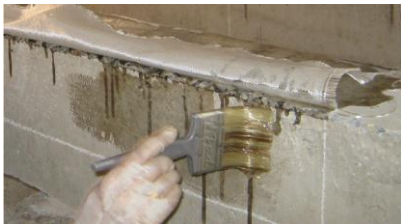
Fig 2. Application of epoxy resin
