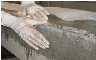
Fig 3 Fixing of GFRP sheet
