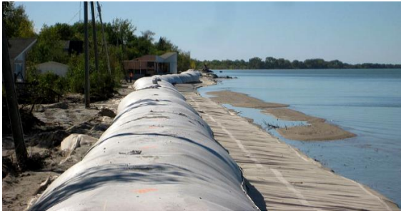
Fig 9: Geotubes on Kerala shoreline
