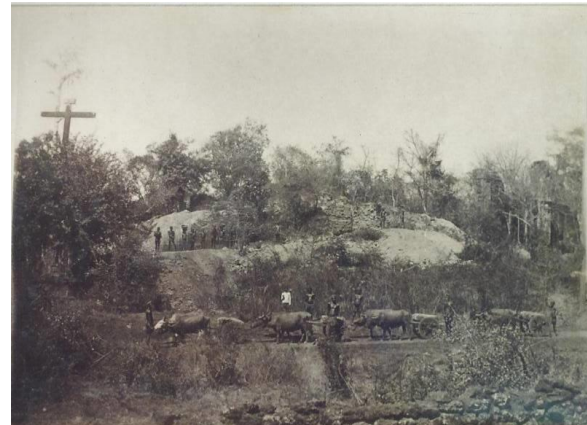
Figure 7: Photo showing moving of material to new city
