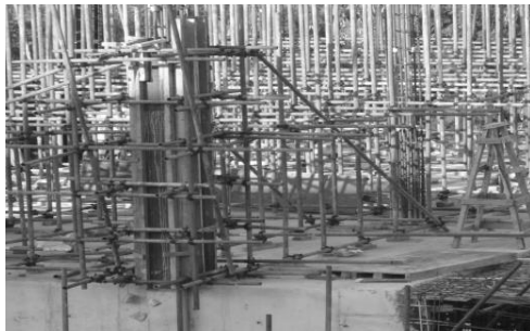
Figure 6 Formwork for a column
