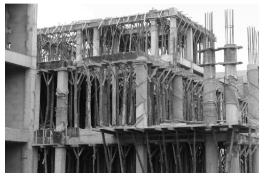
Figure 9 Curing of reinforced concrete members
