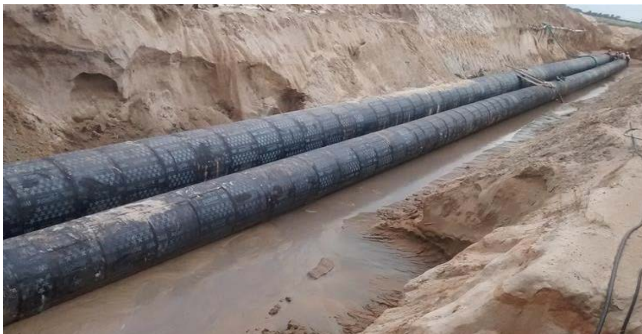
Figure 11: Underground installation of Cooling tower makeup and blowdown lines with wrap coating for external protection.
