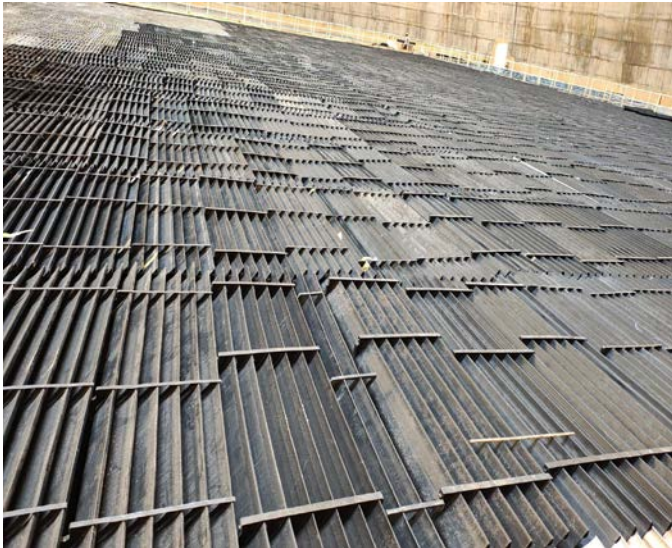
Figure 28: NDCT drift eliminators after repair
