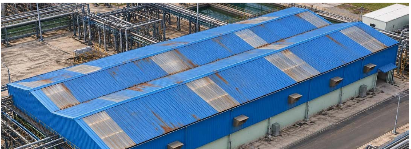
Figure 16: Metal sheet installed DM plant
