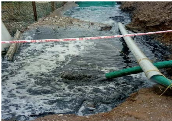
Figure 10: Desilting forebay for removal of silt and barnacles' deposition.
