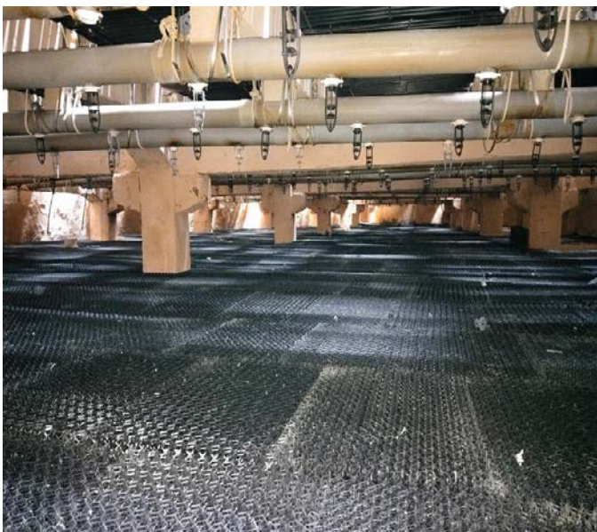
Figure 29: PP fill and nozzles after repair
