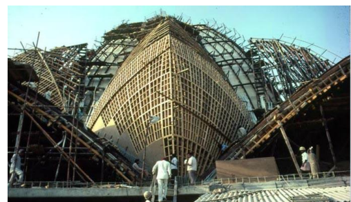
Fig: 11. Formwork
