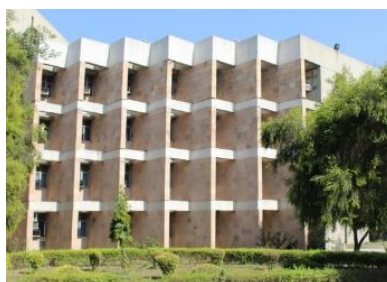
Figure Façade screening through staggered sunshades
