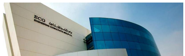
Figure 5. East elevation louvers. (3).
