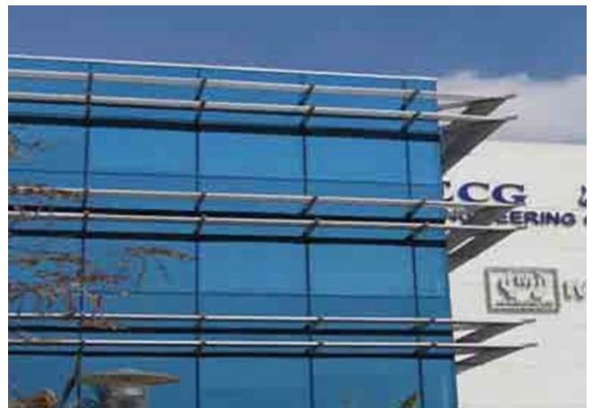
Figure 4. South elevation louvers. (3)
