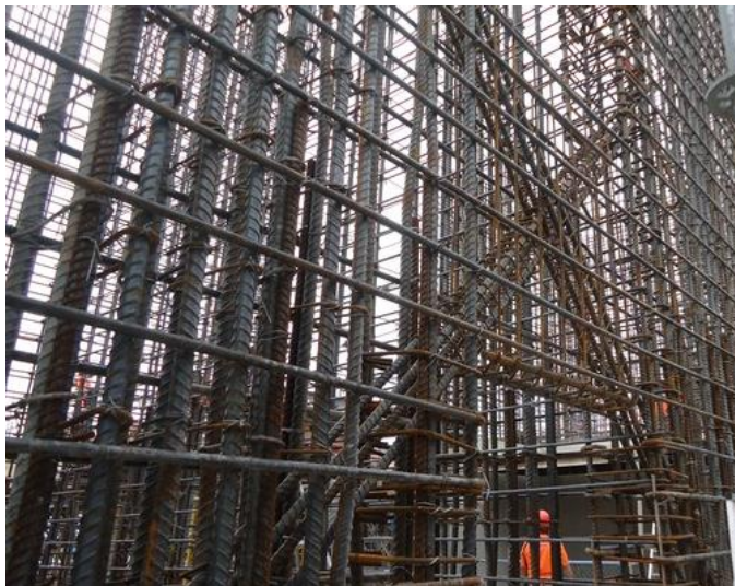
Fig. 3 Diagonal reinforcement in a coupled shear wall
