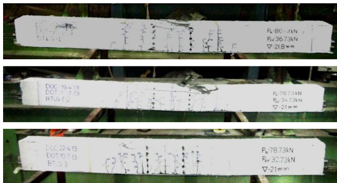
Fig. 10 The cracking pattern of beam BTLG
