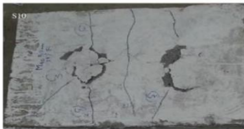
Crack pattern of slab M 40 50mm thickness 1.5% fiber
