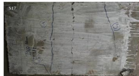
Crack pattern of slab M 60 50mm thickness 1% fiber
