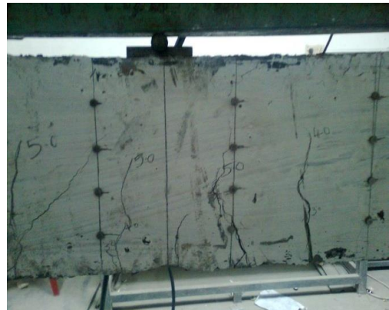
Fig. 2 Showing shear cracks
