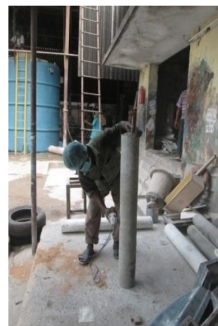
Fig. 2 Removal of loose material
