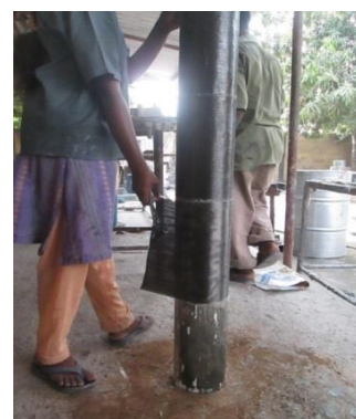
Fig. 4. CFRP Bonding
