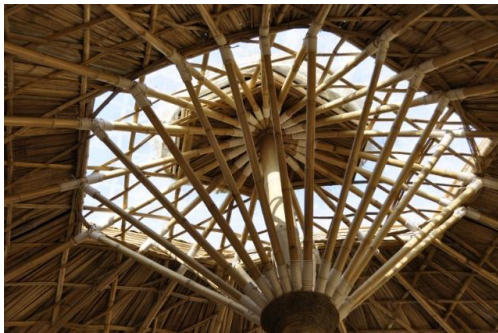
Fig. 8. Bamboo Roof
