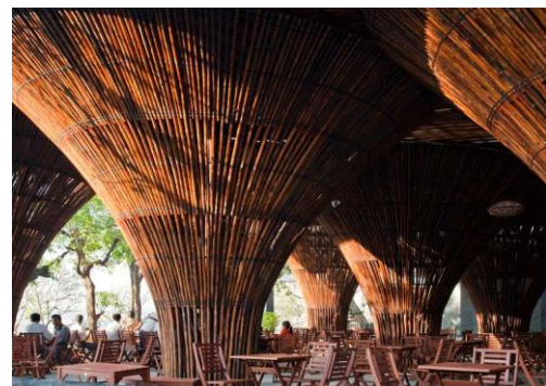
Fig. 6. Layered Bamboo Columns
