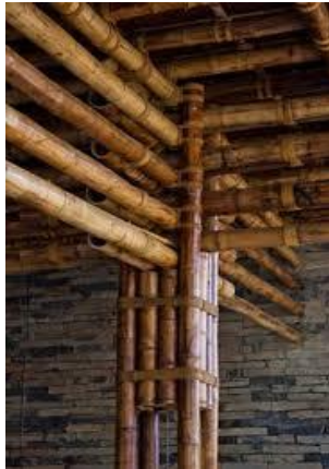
Fig. 7. Beam Column Joint
