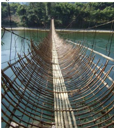
Fig. 3. Hanging Bamboo bridge over Siang River, Arunachal Pradesh, India
