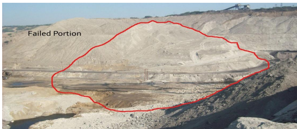
Fig. 1 Failed portion of internal dump slope
