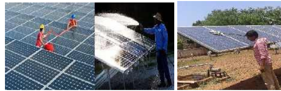
Fig.1.1: Manual cleaning process
