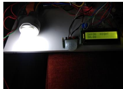
Fig. 8. The load (bulb) is ON
