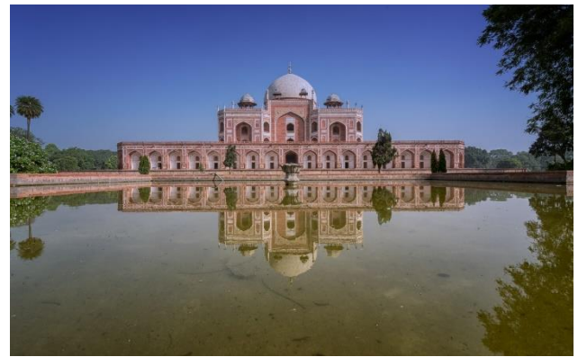
(After) Photo from the central restored water body Photo Courtesy: Photo Artist – © Ar. Vivek Kalla
