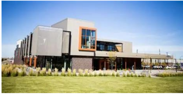
Figure No. 19 Community Centre
