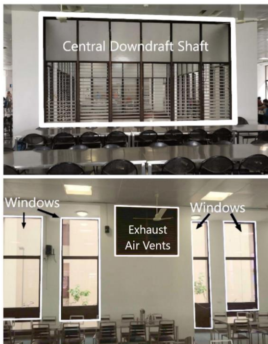
Fig. 3 . Student dining facility: CAD drawing showing plan view of the dining facility and views from inside and outside showing downdraft shaft and exhaust vents (CAD drawing adapted from architectural drawings).
