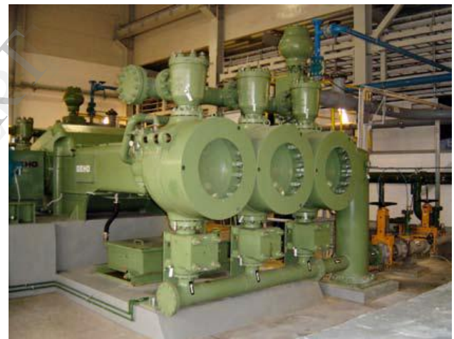
Crankshaft driven piston diaphragm pump
