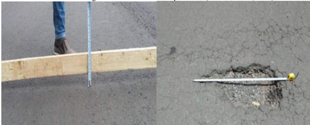
Figure 2: Some sample pavement condition surveys on Shone-Buge subsection
