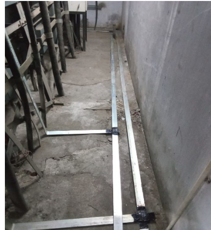
Connect machine and Electrodes through GI Patti
