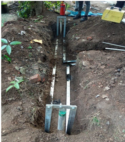
Connect Electrodes through GI Patti
