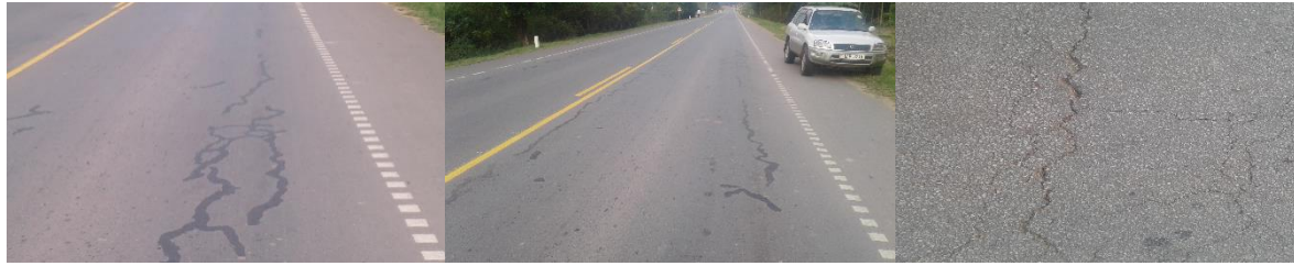
Northern Corridor Route, Lot 1 Northern Corridor Route, Lot 2 Northern Corridor Route, Lot 3
