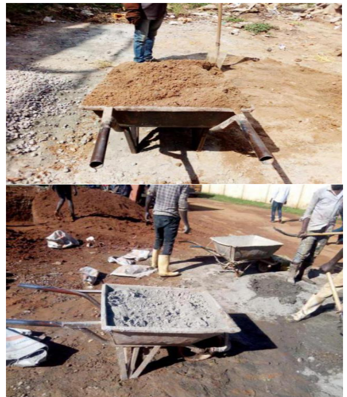
Figure 1 : Wheel barrow full of sand and wheelbarrow of cement (50 kg bag cement)
