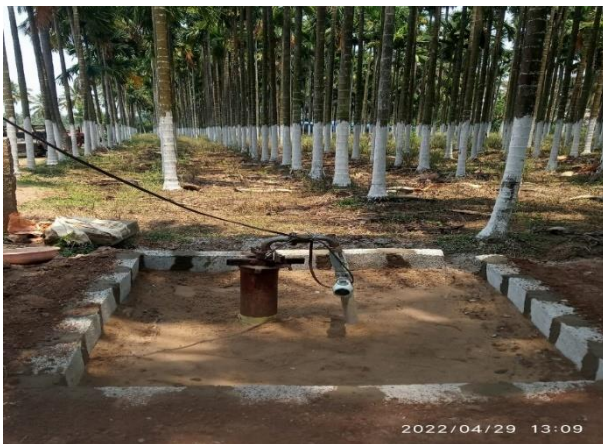
Fig 10: Protection wall for ponding water.
