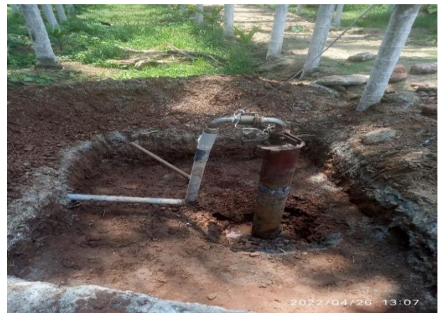
Fig 3: Excavation of recharge pit.
