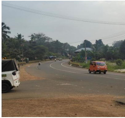
Fig. 5 Road bend contributing to increased collision possibility
