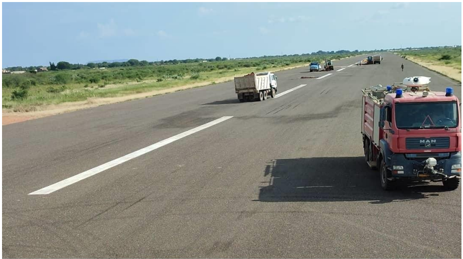
Figure 5: applying the maintenance in runway
