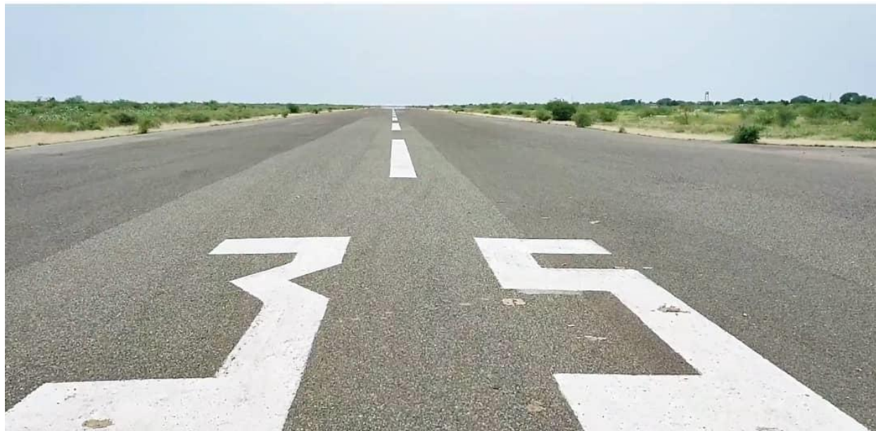
Figure 7: added signs to the runway after the maintenance completed
