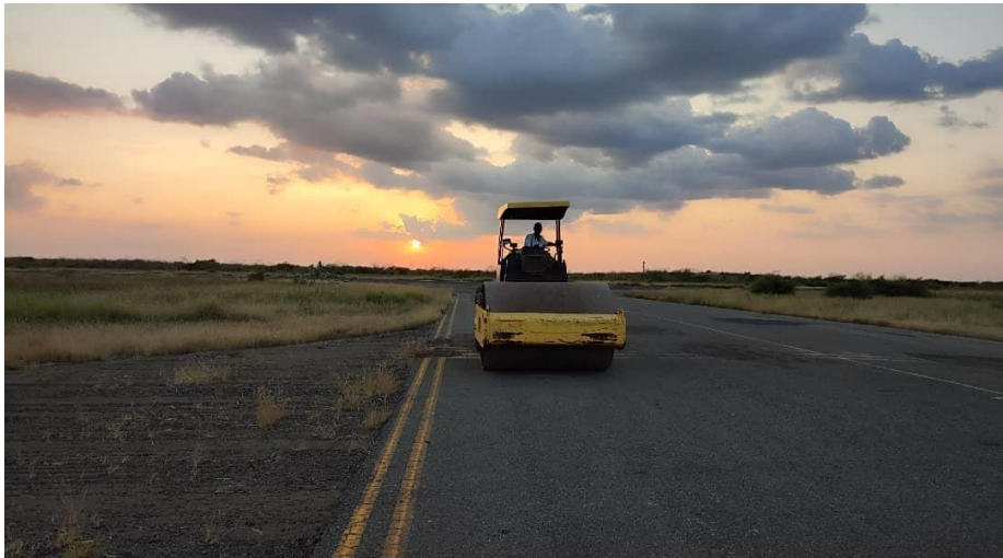
Figure 6: the compaction to treated pavement to the top surface
