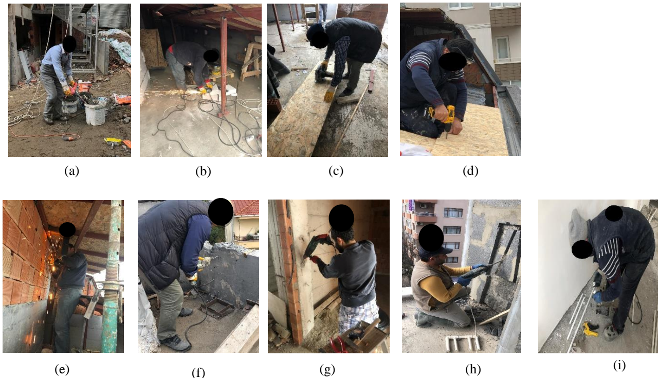
Fig. 2. a) Plaster mortar preparation process b) Metal cutting process c) Die cutting process d) Roofing process e) Welding process f) Concrete crushing process g) Drilling process-I h) Drilling process-II i) Plumbing process
