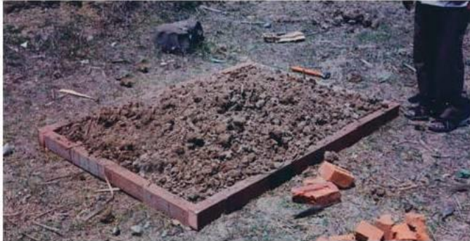
Photo 1: Making of mould 2.5m x 2.0m
