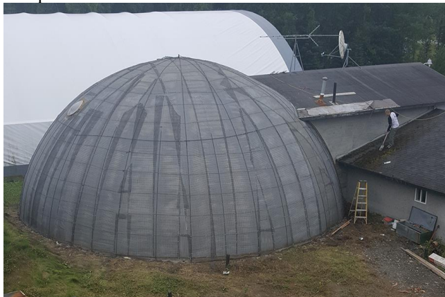
Fig 6. Domes with basalt mesh in Soldotna
