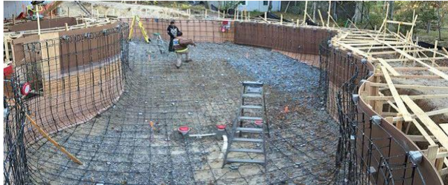
Fig 1. Swimming pool constructed with basalt rebar
