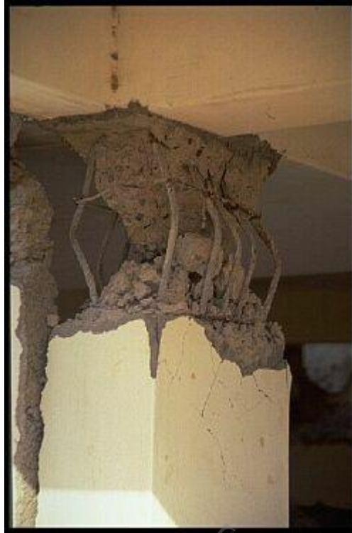
Figure 1a Damage to columns in sabthagiri apartment.
