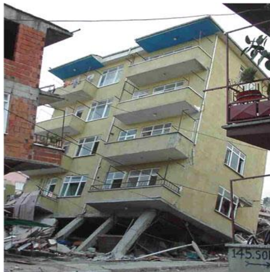
Figure.1b Soft story failure, Bhuj 2001
