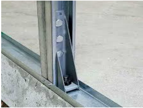
Figure1.5: Typical Hold-down Members
