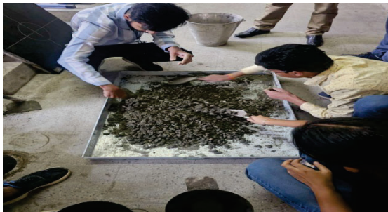
Fig.1 Mixing of concrete
