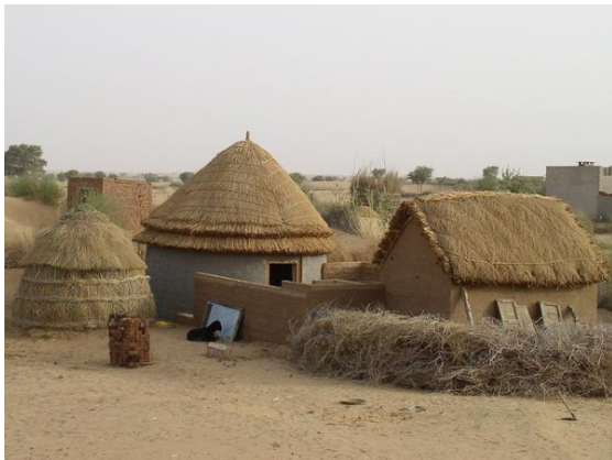
Fig.12.Mud-Cement Stabilized New Houses in Barmer District[19]
