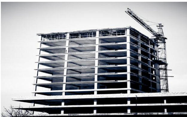
Figure 1.1 Conventional frame building
