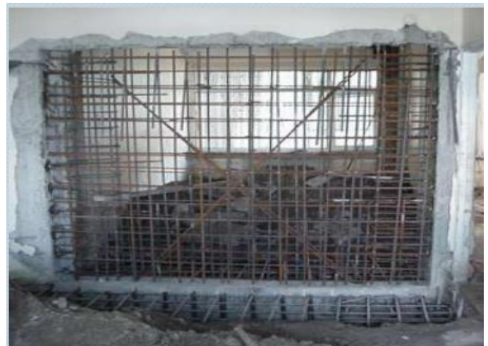
Fig. 2: Additional shear wall
