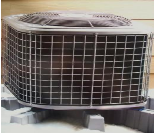
Fig no.2.2 The condenser in a central air system.
