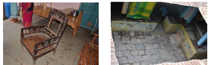
Fig.12 Floors of Verandah & Courtyard
