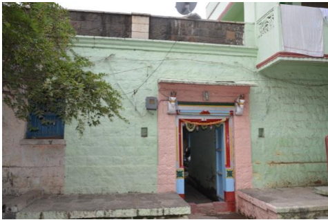
Fig.3 Main Entrance of the House
