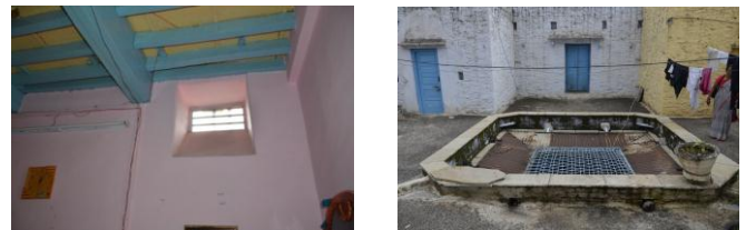
Fig.13 Ventilator & Shading device
