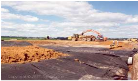
Fig. 2 Example of an woven geotextile material
