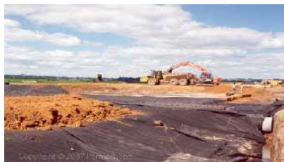
Fig. 1 Example of an non woven geotextile material
