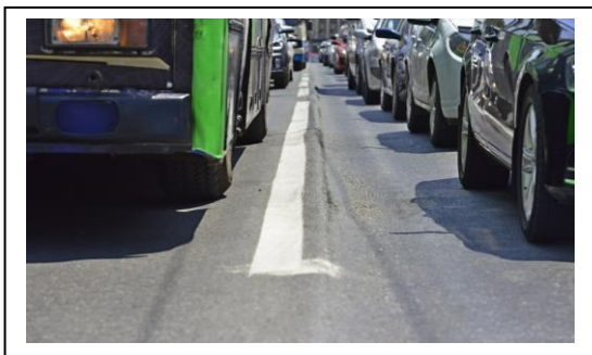
Figure 1. Typical rutting development in asphalt pavement subjected to repeated stopping and standing loads of public transport vehicles
