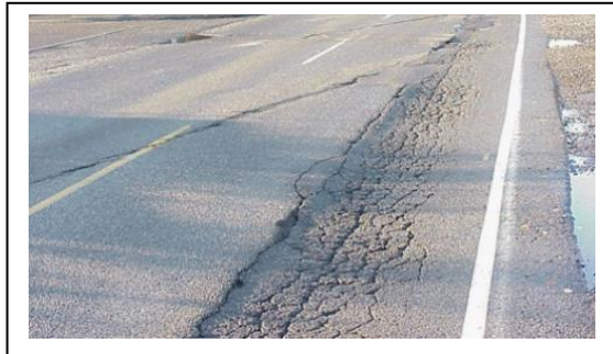
Figure 3. Typical rutting and shear-related surface deformation observed in asphalt pavements subjected to repeated stopping and braking loads in urban public transport stop areas [1]
