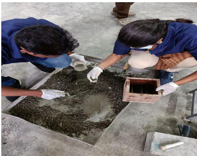
Fig 9: Placing first layer of concrete mix
