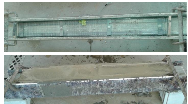
Fig.7 grouting steel wire mesh jacket using Cetorex grout
