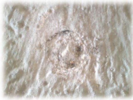
Fig 8 Initial failure on specimen
